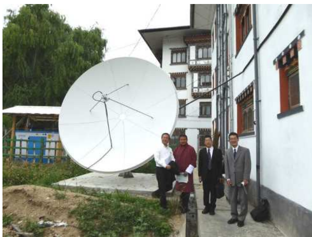
Figure 2. 3.4m-diameter antenna at DHMS
