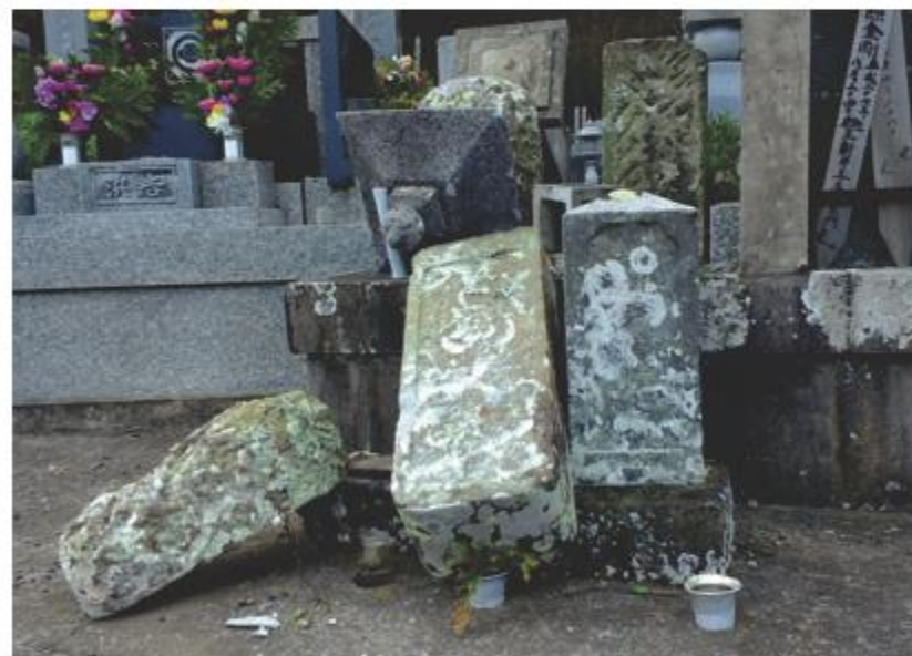
DI 27: Gravestones DOD 1: Slip or Overturning (LB 45m/s) (Minami-Boso City, 22 August, 2016)
