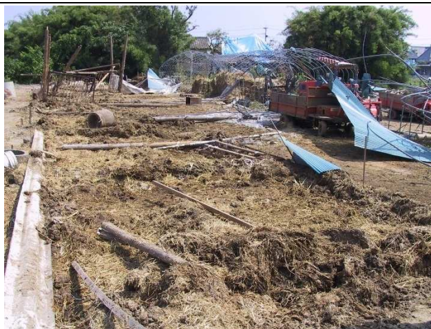
DOD = 5 Major deformation/collapse of upper structures
