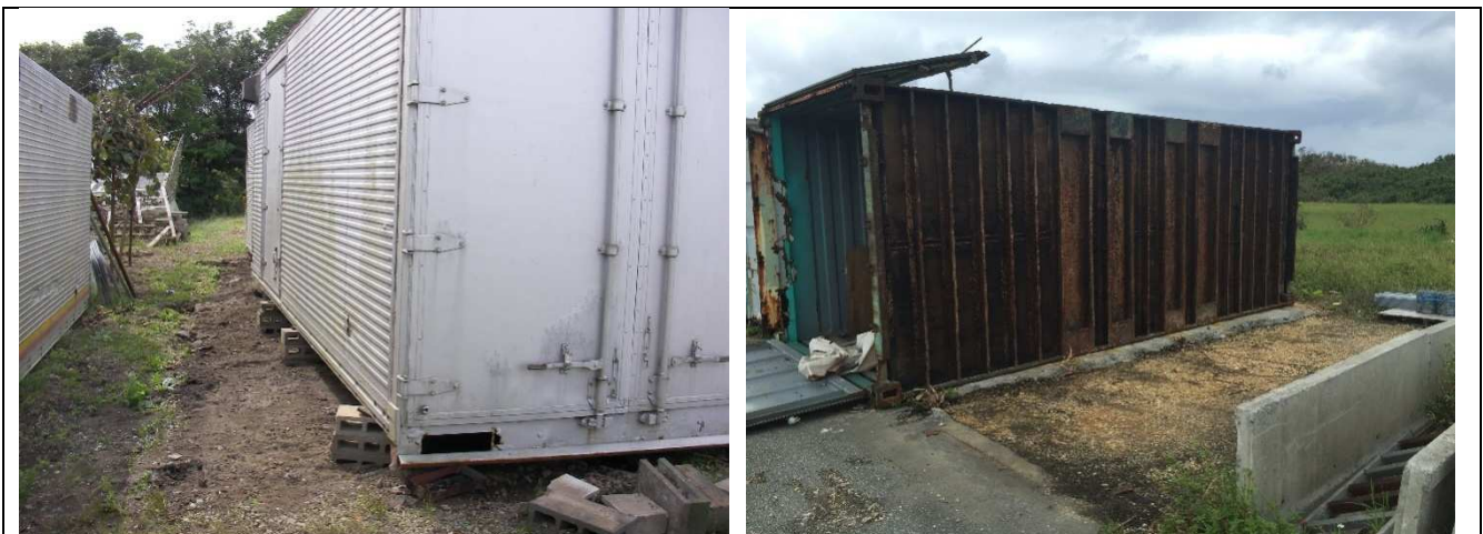
DOD = 1 Slippage/overturning with content of 0 – 300 kg Container slippage (left) and overturning (right)
